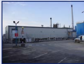
▲ Page 2 Total Substation
